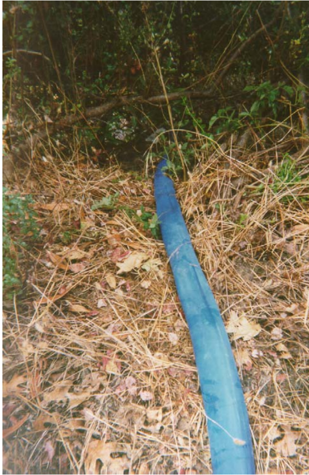
Discharge to Vegetated Area at PRIV-10
