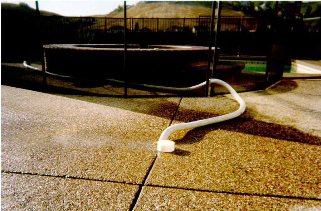
Discharge into Storm Drain at PRIV-11
