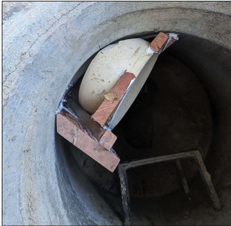
Figure 5. Ohlone Greenway Influent Pipe Extension
