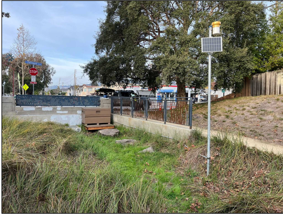
Figure 3. Ohlone Greenway Equipment Installation
