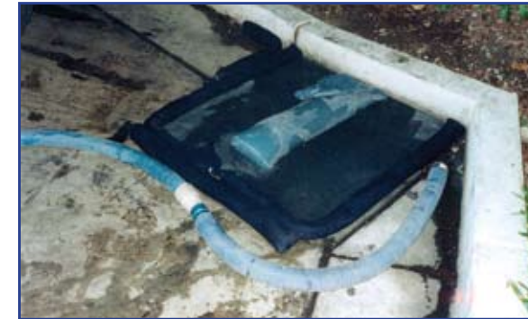
A storm drain cover with vacuum hose.
