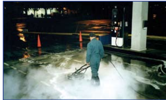
Spinner cleaning a gas station, to collection system.
