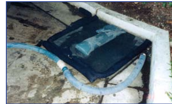
A storm drain cover with vacuum hose.
