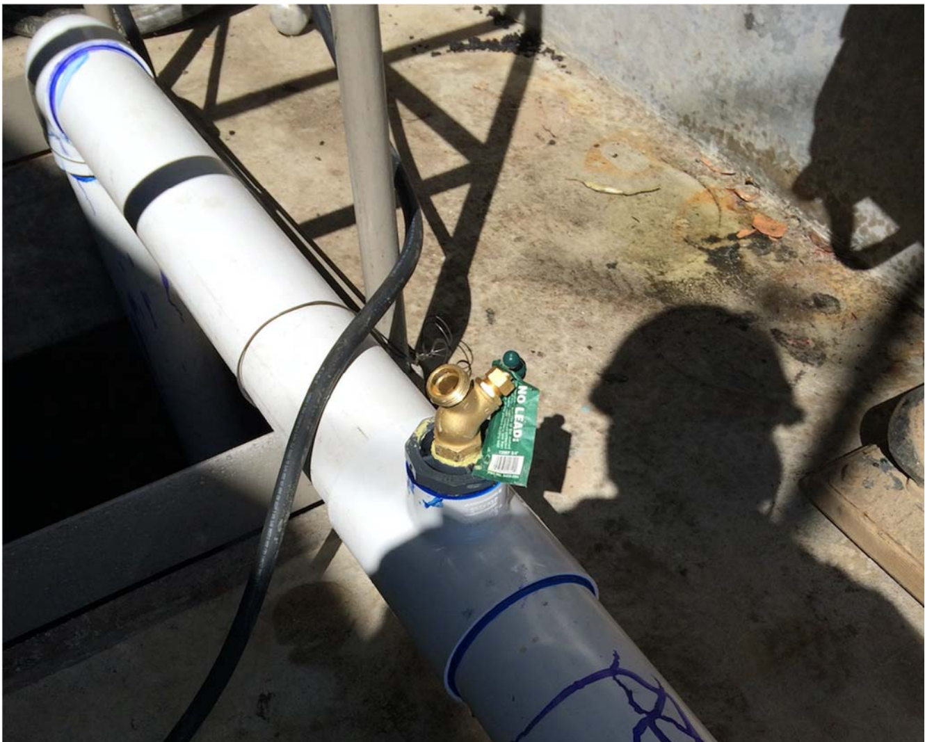
Figure 1. Monitoring Spigot at Diversion Pipe
