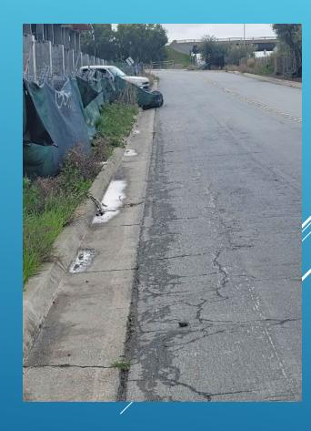
Failure to maintain these BMPs was causing significant amounts of sediment laden discharge along with sand bag material and plastic. This also was causing the discharge pipes to clog flooding the street during heavy rains.
