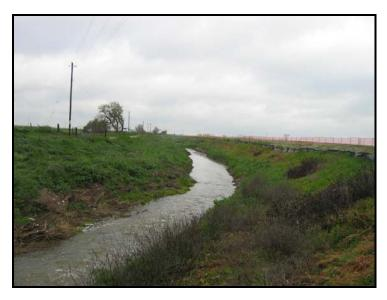
**SITE NOTES:** Trapezoidal channel confined within constructed levees. Well vegetated. Minor internal meandering within levee caused by localized point bars. Terrace formed within levees implies excess capacity within the levee. Simplified channel morphology. Cohesive clay substrate with limited non-cohesive sediment in transit.
