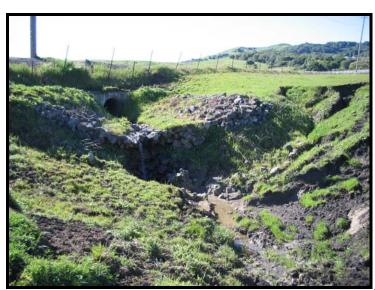
**SITE NOTES:** Massive degradation of channel due to incision and destabilized bank failures under existing land-uses. Degradation partially due to poorly designed and/or maintained infrastructure.
