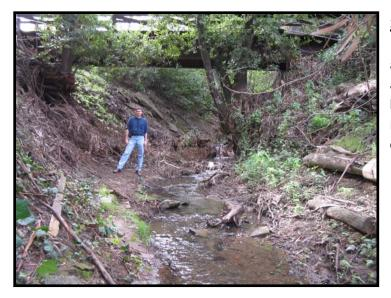
SITE NOTES: Channel incised about 15-18 feet into a small, confined valley along older sub-division. Road is adjacent to channel. Clear signs of bank instability evident through informal hardening efforts (e.g. brick, old asphalt, log revetments etc.).
